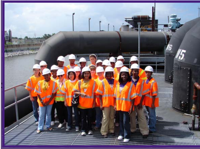
2008 REHAMS and XCITE camp participants during a tour of the 17 th street canal pumping station
